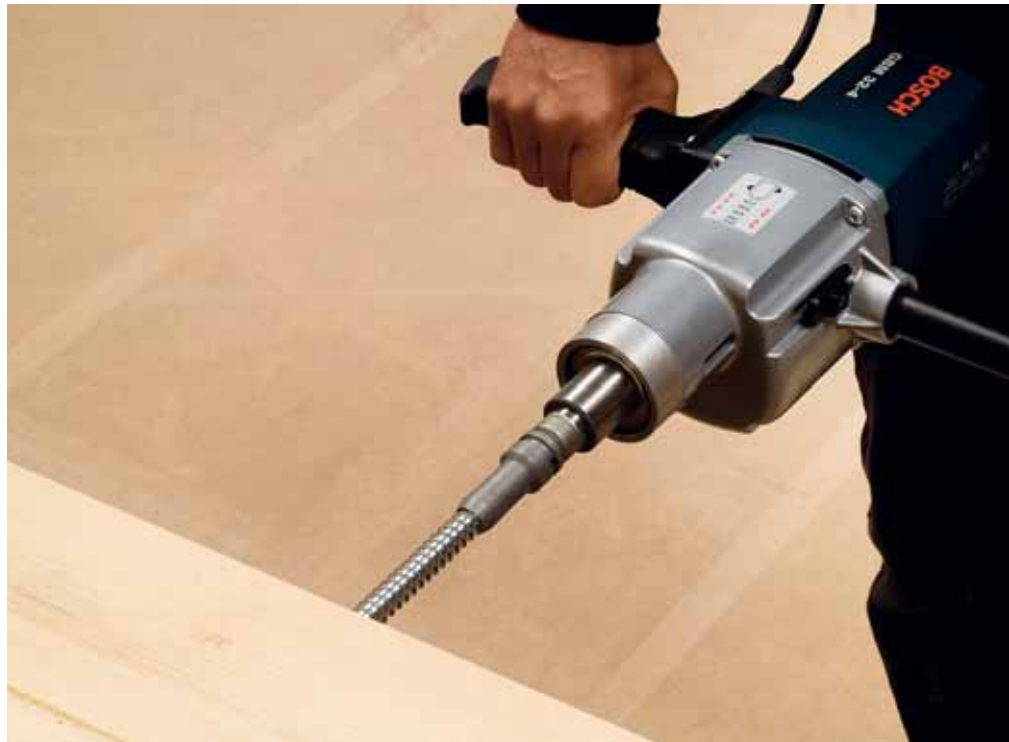
4. Install the threaded bar using a drill with high torque.
